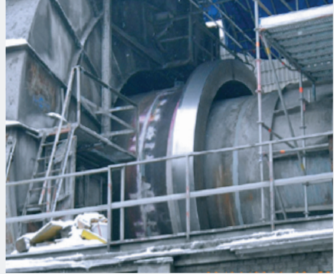
Station IV of a rotary kiln with planetary cooler
