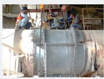
Damper during installation into a horizontal piping section of the tertiary air duct.
