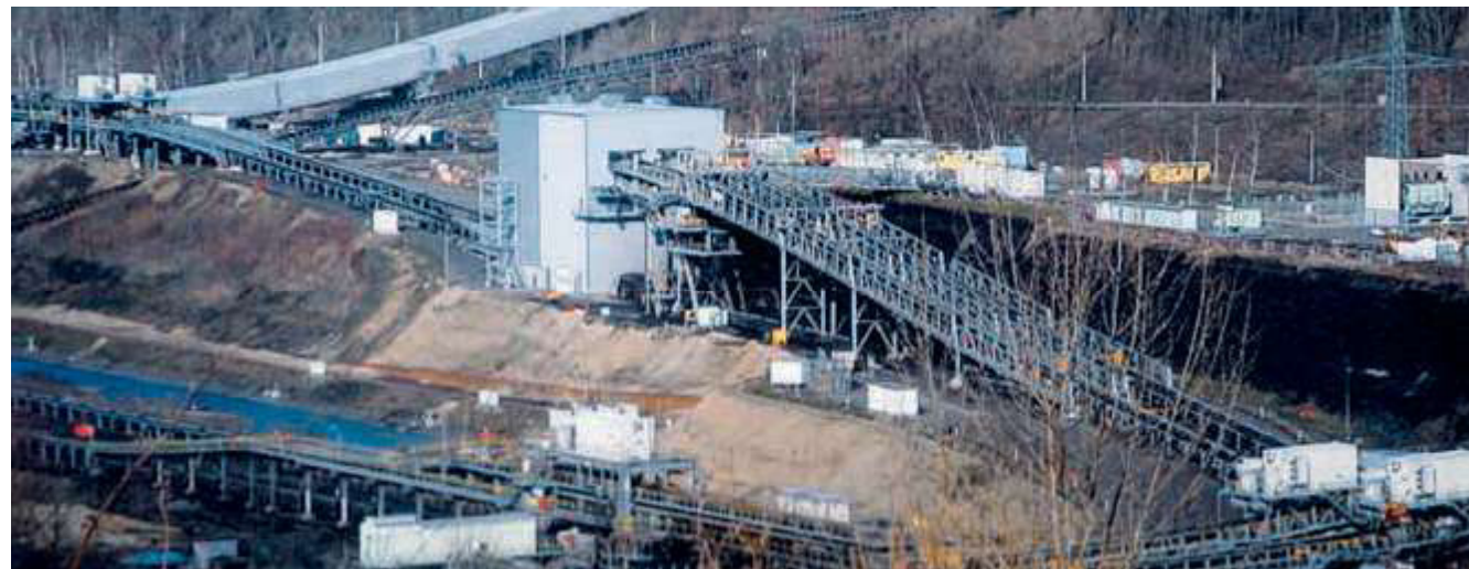
Lignite processing plant built by thyssenkrupp Industrial Solutions with four RollSizers, DRS 660 x 3700 SideSizers, in operation.
