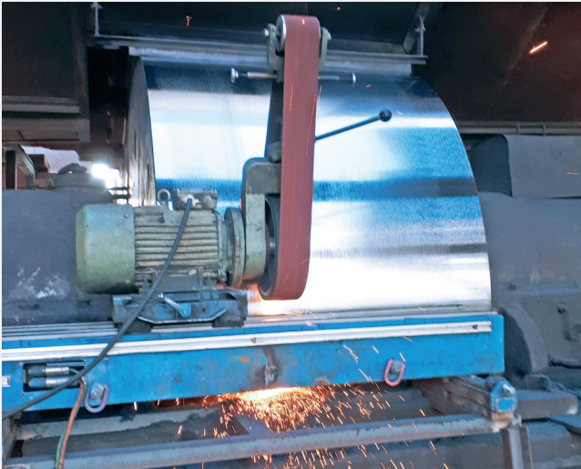
Grinding work on the tyre and a supporting roller
