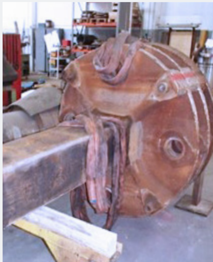
Rotor refurbishment in the Service Center Münsterland
